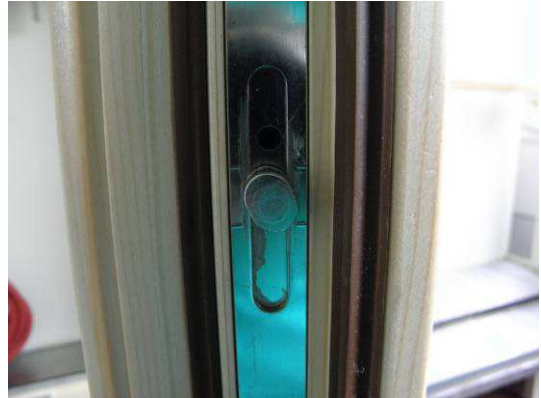
Picture 34 Locking situation, frame member / casement member 3
