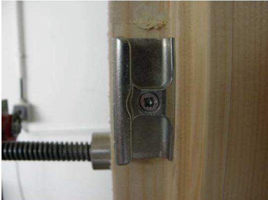
Picture 33 Locking situation, frame member / casement member 3
