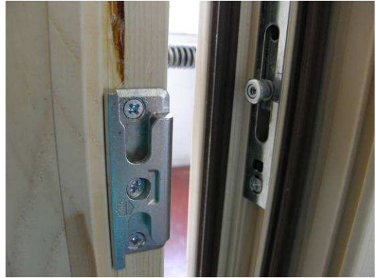
Picture 32 Locking situation, frame member / casement member 2
