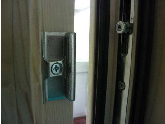
Picture 31 Locking situation, frame member / casement member 1
