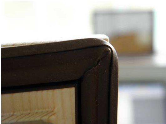
Picture 17 Internal rebate seal, corner configuration
