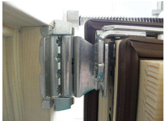
Picture 28 Tilt mechanism pivot, rebate view
