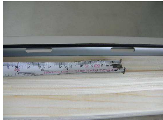
Picture 4 Rebate drainage
