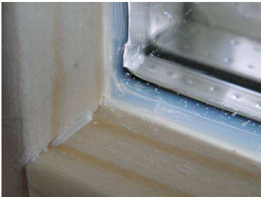
Picture 21 External glazing seal, corner configuration
