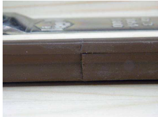
Picture 16 Centre seal, sealant joint
