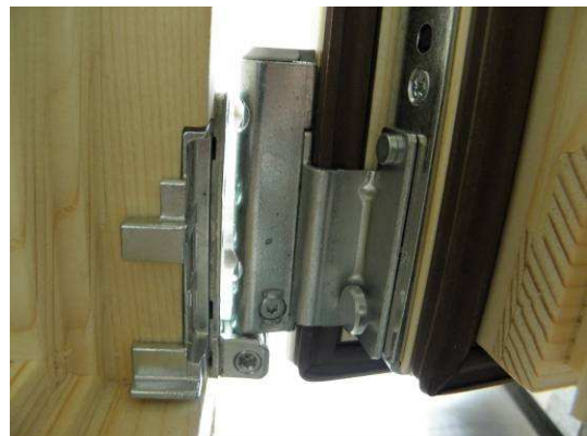
Picture 30 Corner pivot, rebate view
