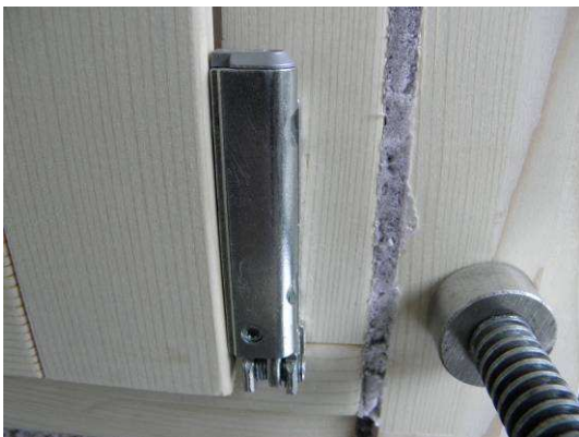
Picture 29 Corner pivot, internal view
