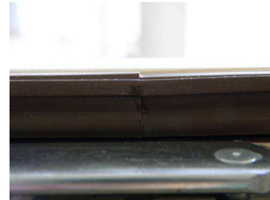
Picture 18 Internal rebate seal, sealant joint
