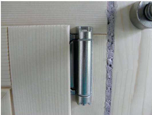
Picture 27 Tilt mechanism pivot, internal view
